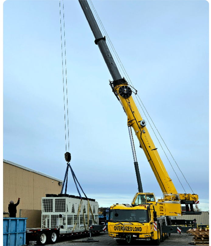
Pre-piped skid being installed
